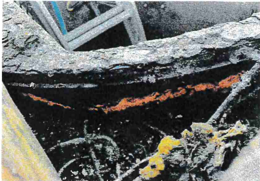
EXTERNAL OF FIBERGLASS STORAGE SHOWING THROUGH WALL SUNLIGHT
