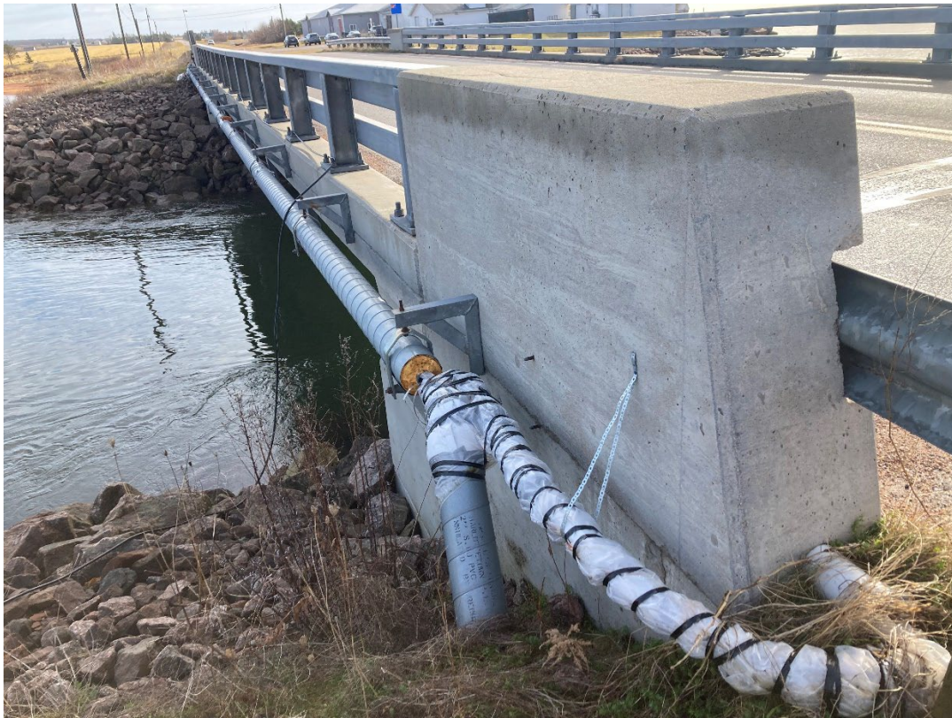
Figure 1.0 – Existing Temporary Watermain Repairs
