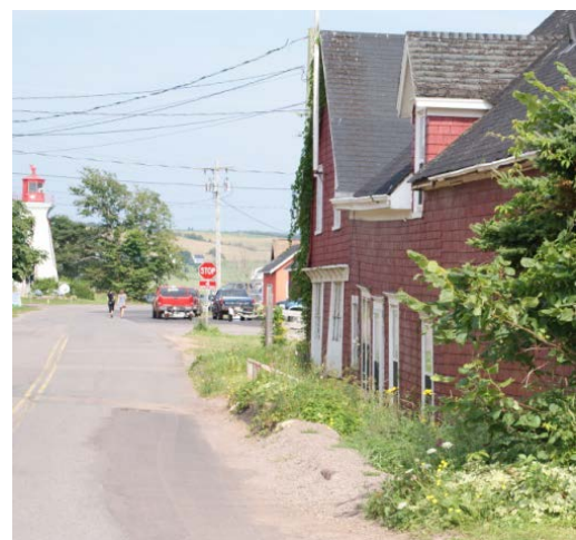
Figure 5 - Main Street has been raised and is now higher than homes on the south side of the street (photo credit: P. Nishimura).
